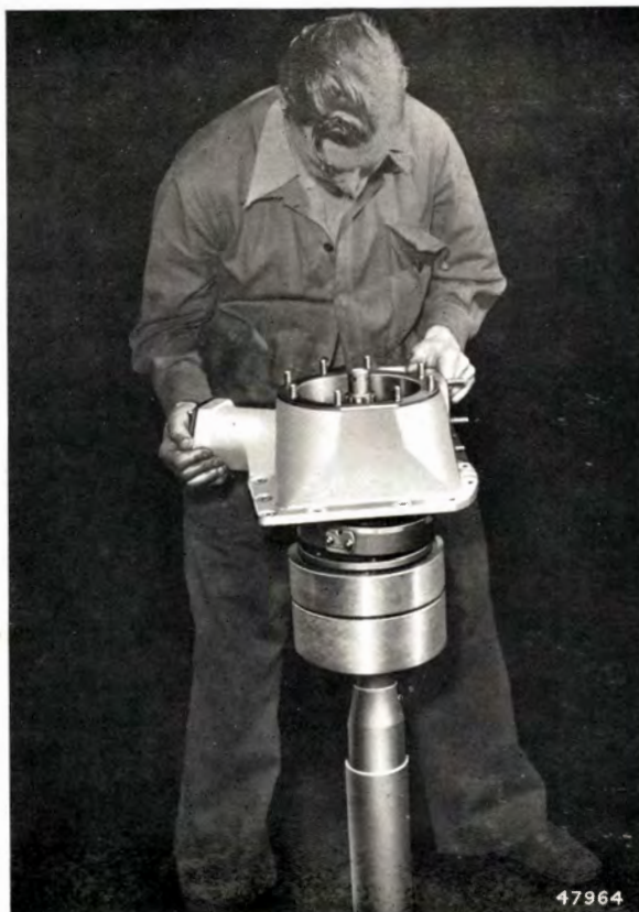
FIG. 38. FITTING THE FRONT COVER ASSEMBLY
